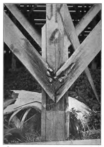
Fig. 34.—Decay in braces at a joint where moisture has collected.
